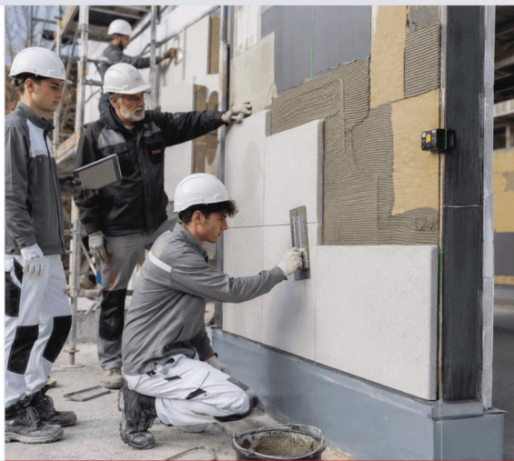
Facade insulation and finishing practice in a vocational workshop.
