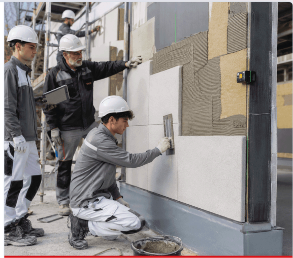
Facade insulation and finishing practice in a vocational workshop.
